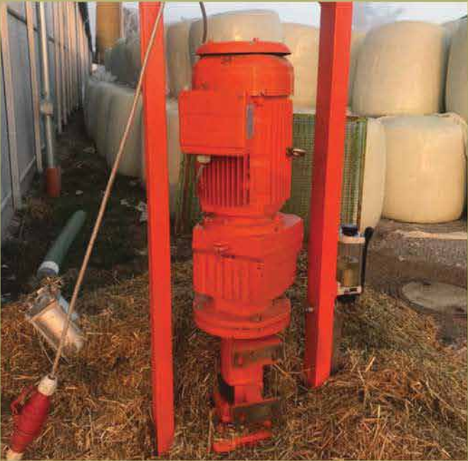
LIQUID MANURE PUMP Flow – 40 m³/hr, Pressure – 4.5 bar
