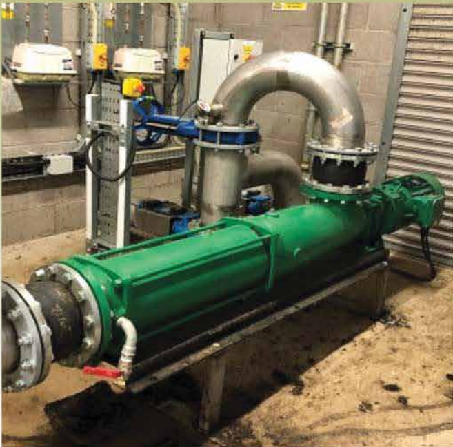
BIOMASS RECIRCULATION PUMP Flow – 80 m³/hr, Pressure – 4 bar
